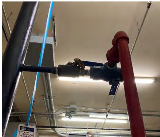
Valve in relief flow path not permitted by CSA B52
