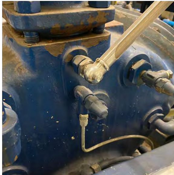
Needle valve not permitted by CSA B52
