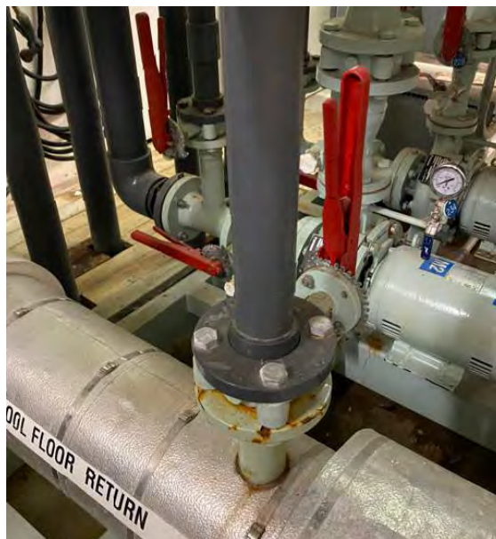
Expansion tank valves with no administrative control present on valve handle
