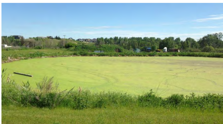
Figure 4-7 Excessive Algae Growth in Polishing Cell
