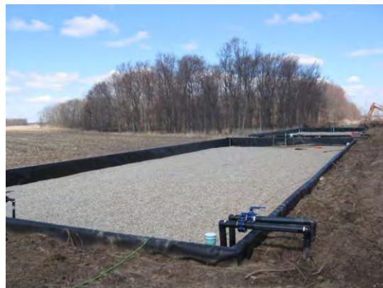
Figure 5-7 A SAGR System in Construction
